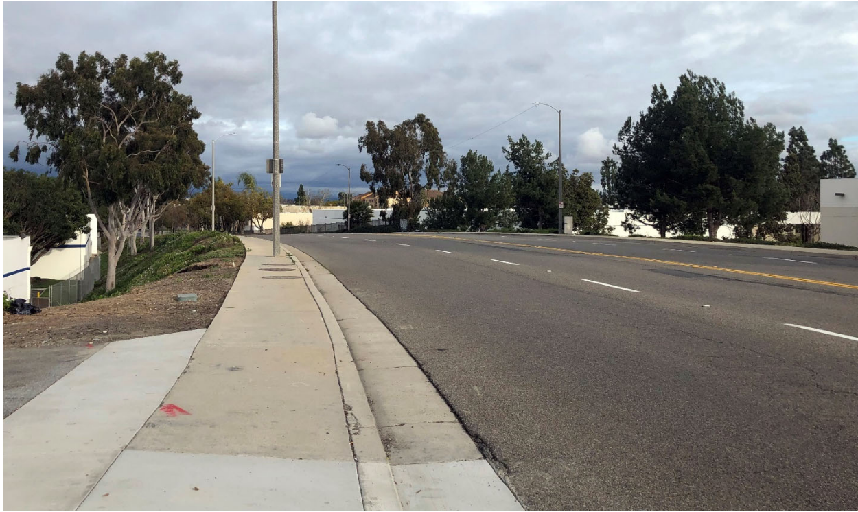
Image 9: Sidewalk with No Buffer Adjacent to Travel Lane
