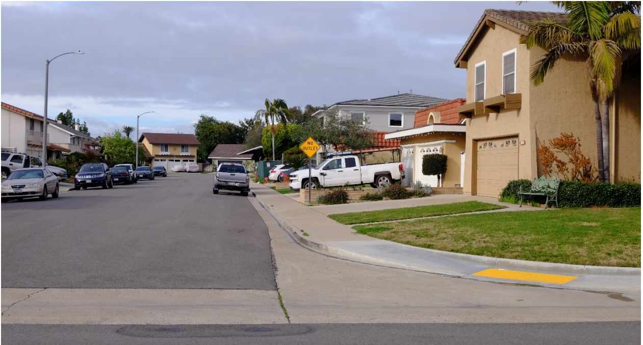
Image 1: Sidewalk with Accessible ramp
