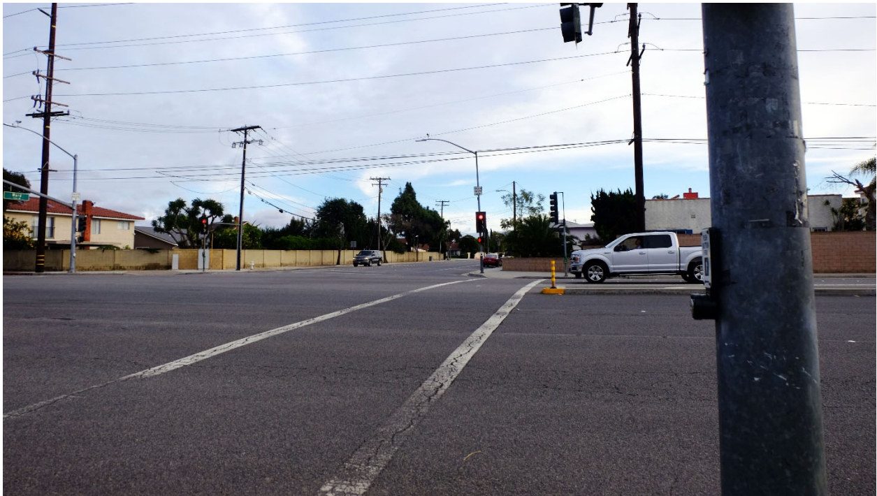
Image 5: Aging Crosswalk Infrastructure Sidewalk in image is located at Warner Avenue and Ward Street
